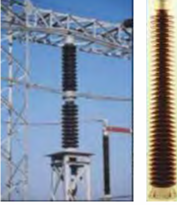
YG Mesnet İzolatörleri/ HV Support Insulators.
